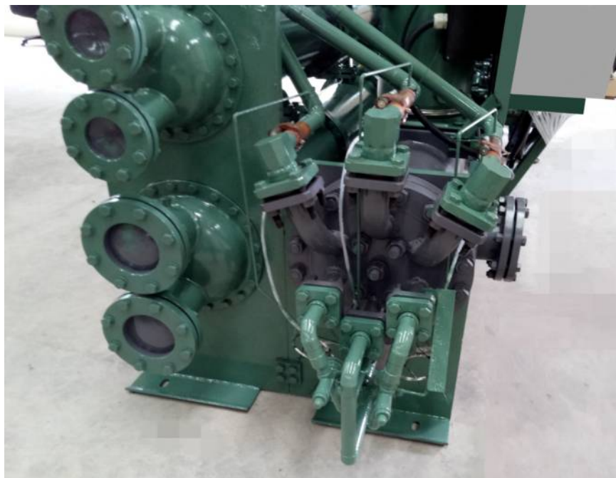
COMMON WATER CONNECTIONS FOR CHILLER AND HOT WATER
